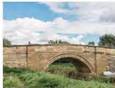
Strensall Bridge – Sheriff Hutton Road
