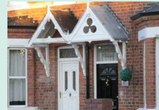
Photo 45: View of decorative detailing
