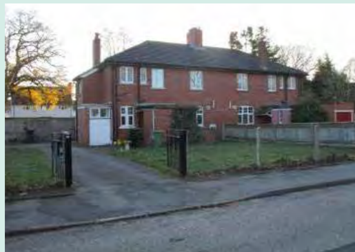
Photo 16: Housing on south side of Alexandra Road
