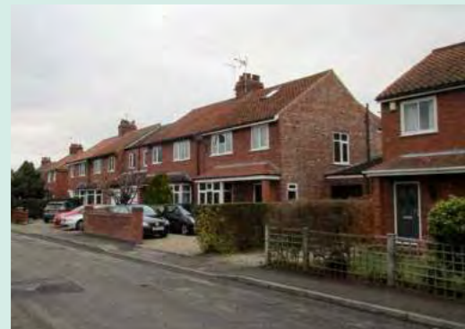
Photo 25: Housing on Moor Lane
