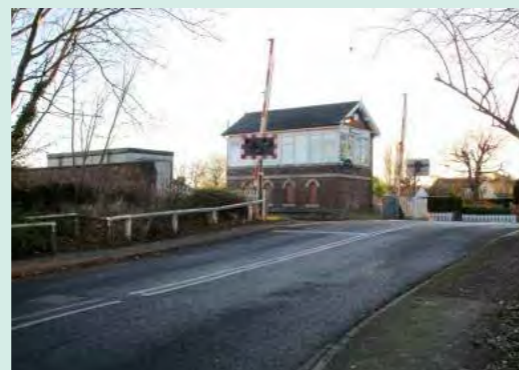
Photo 10: Level crossing at Lord's Moor Lane
