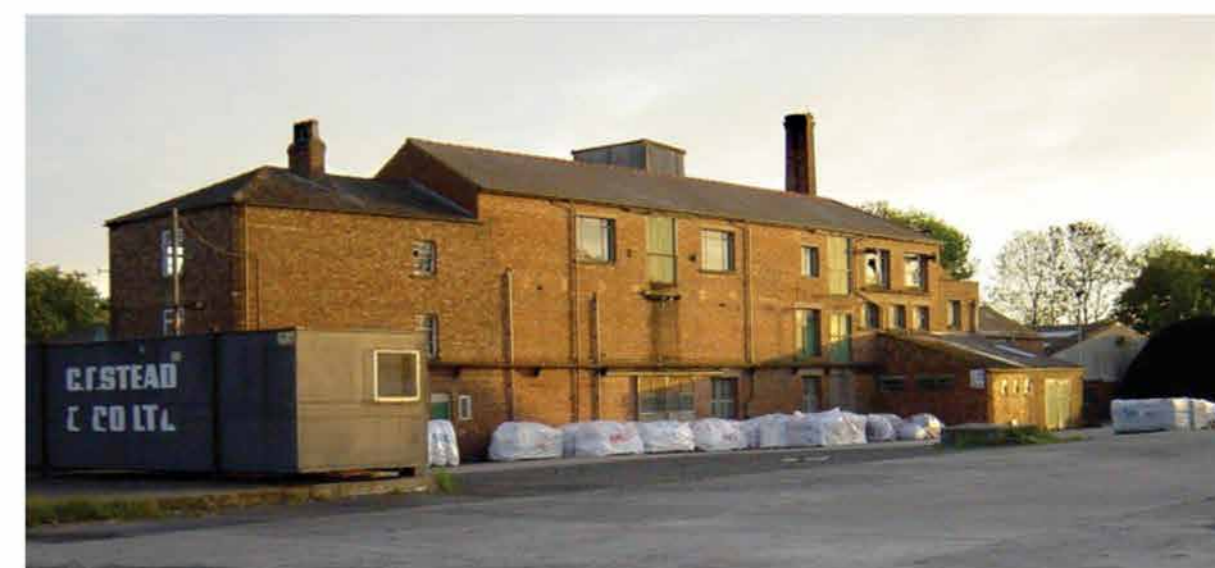
The Tannery, Strensall, now demolished
